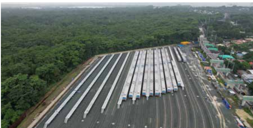
MRT-7 - Depot Facilities, Manila, Filipinas
